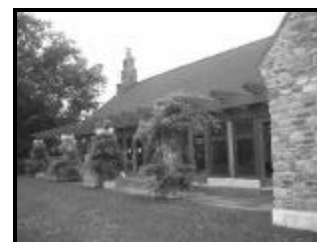
St. Columba's Parish Center
